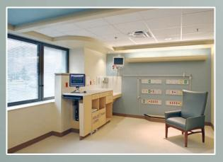
**Provide Comfort** in small spaces where glare from direct down lights can be unpleasant and disconcerting. The CLC Cove System on the wall provides soothing, indirect light in the NICU exam room pictured. The cove system combines wall mounted, eight foot sections of decorative cast GRG (Glass fiber Reinforced Gypsum) cove with a high performance lighting component. Molded castings cut labor costs and can be customized.
